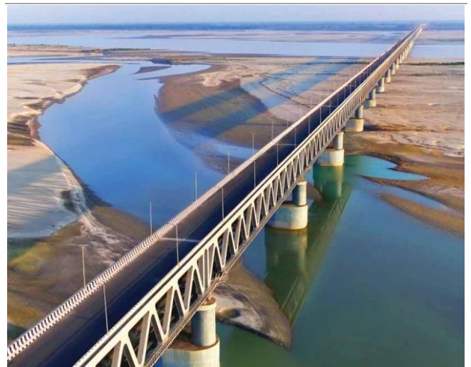
Exhibit 11: 4.9-km-long Bogibeel Bridge in Assam
